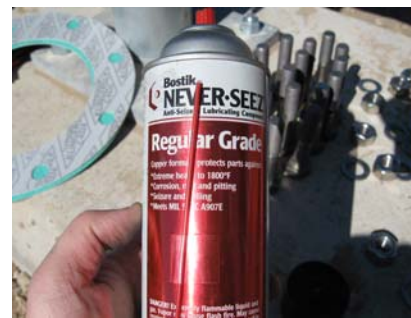
Reverse the process for reinstallation. Use new seals and Never-Seez on the stainless steel bolts and seals.
