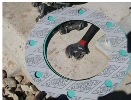
Reverse the process for reinstallation. Use new seals and Never-Seez on the stainless steel bolts and seals.
