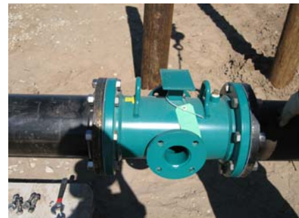
Flow Tube does not leave the process. Sensors, coils, electrodes and grounding rings removed
