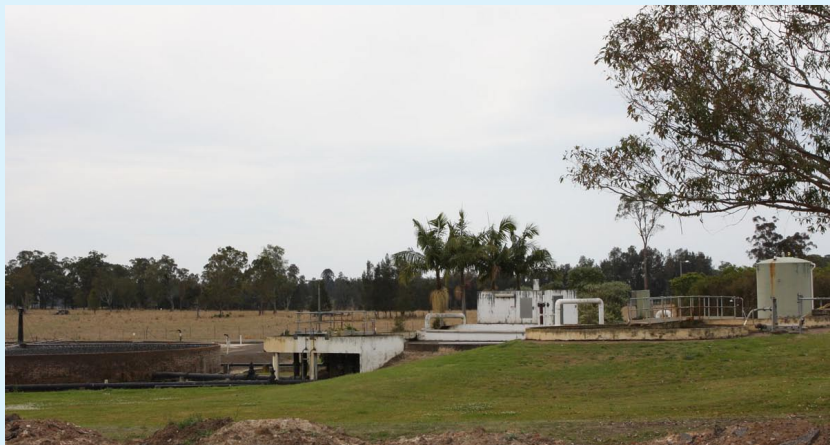
Figure 2: A Typical Mid North Coast sewer treatment plant (STP) near Kempsey, NSW.
