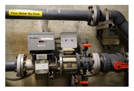
B) Four (4) Toshiba Density LQ meters from the sludge thickener to the sump. -Photo of Armondo Suarez Jr.
