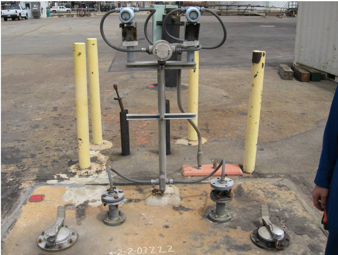
Leaking valve assembly through packing, replace with BAT probe and assembly
