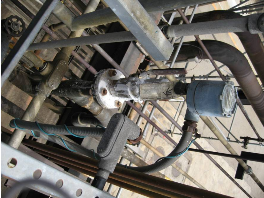
Leaking valve assembly through packing, replace with BAT probe and assembly
