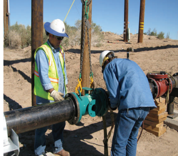
Installation of EMCO Unimag
