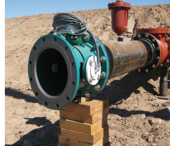
12 Inch mag installation
