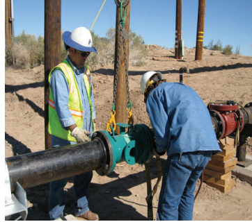
Installation of EMCO Unimag
