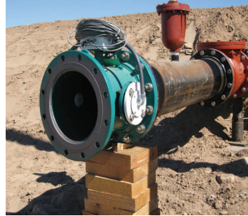
12 Inch mag installation
